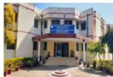
CSB-RSRS, Sahaspur (UK)
